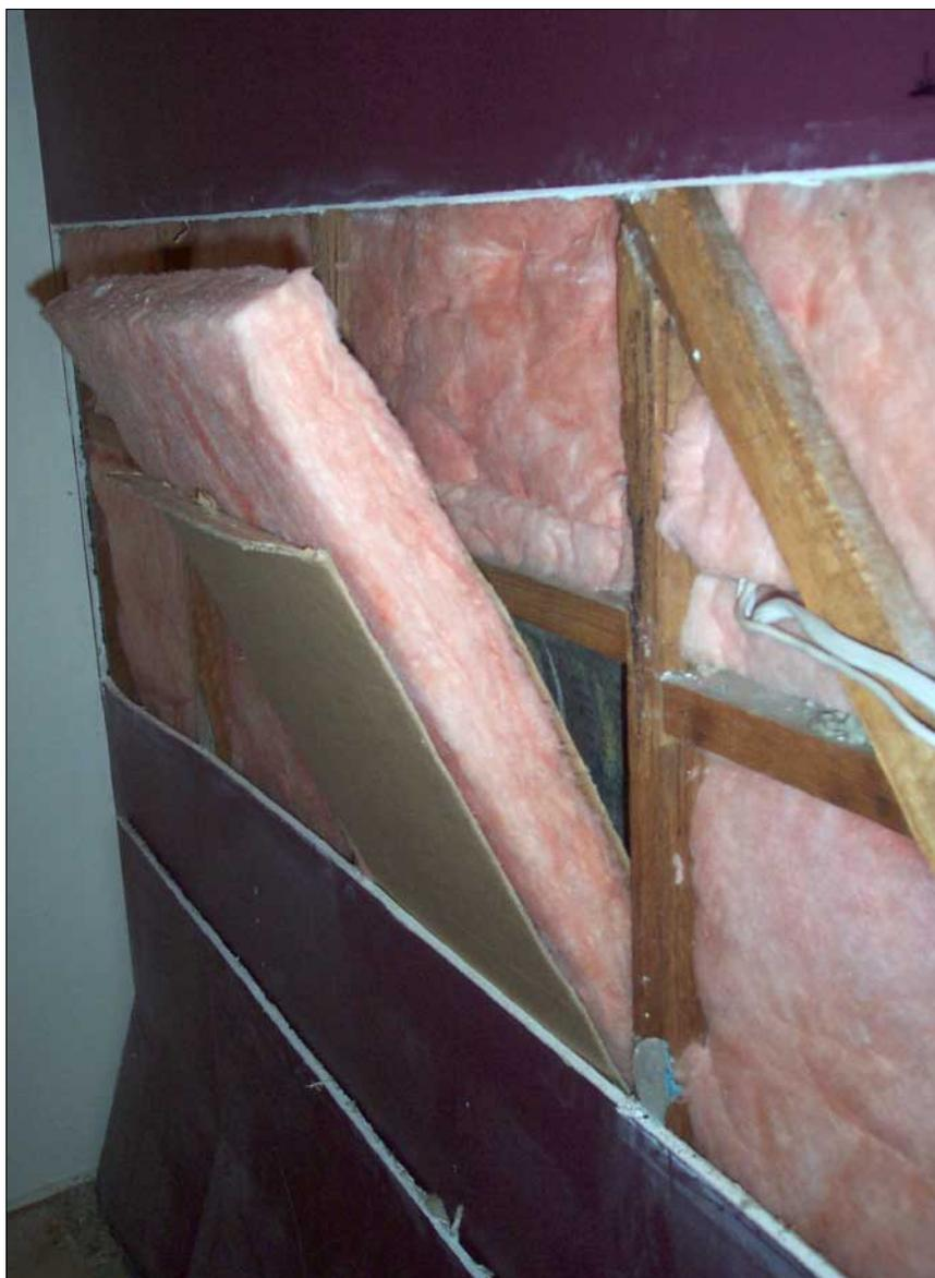
Sliding a batt into the wall. The cardboard either side of the batt makes this much easier, and eliminates the risk of coming into contact with exposed wiring.
