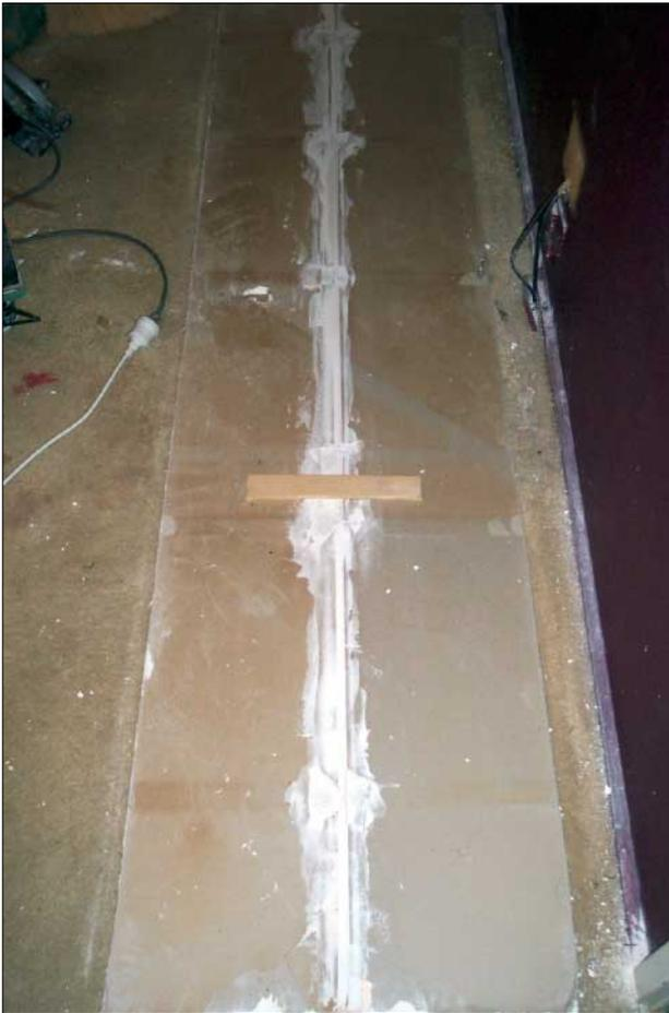
**Bracing and patching the plasterboard strip before replacing it.**
