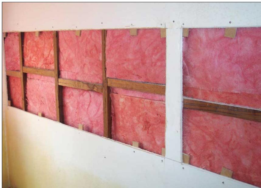
The plasterboard is cut into two sections to make them easier to handle. Small blocks of MDF are used to stabilise the new joints and screws fixed to keep the existing plaster in place.
