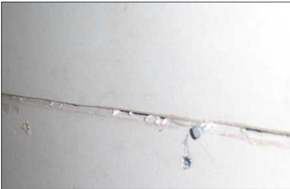
The photo shows the old nails used to create a gap, with some jointing plaster in place before the board was fixed into place. Note the extra screws used to fix the existing plasterboard firmly to the studs to minimise forces on the joint over time.
