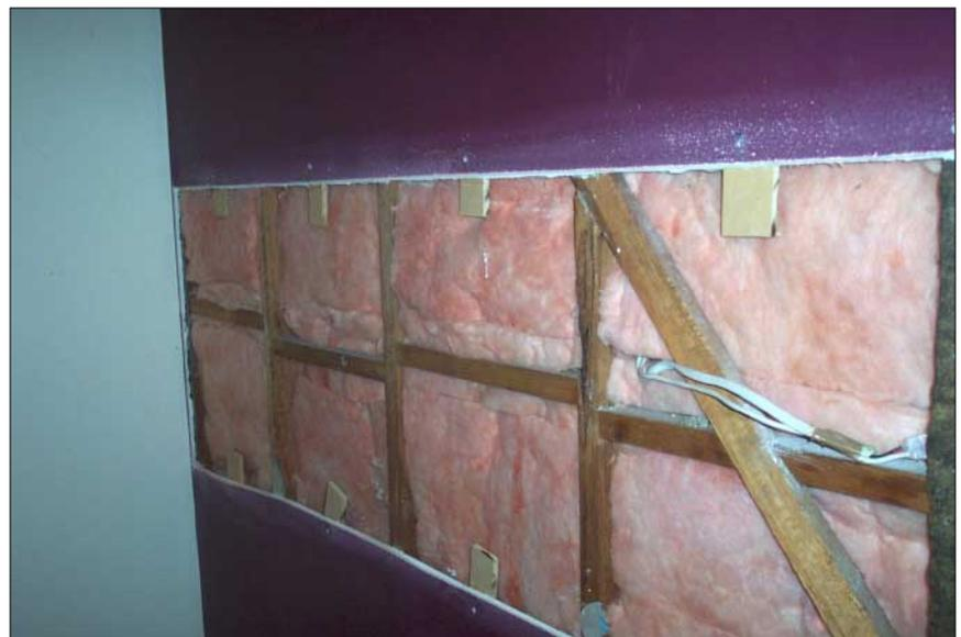
After the insulation is installed. Note the small pads to support the plasterboard when it is replaced.
