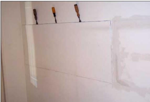
A number of chisels and strips of metal were used to gently lever the plasterboard off the wall without breaking it.
