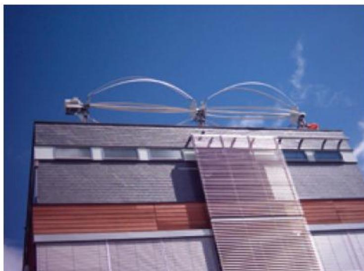
**Figure 2.15:** Windwall turbine in the Hague
