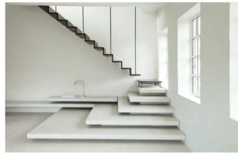
This dramatic staircase is part of a Copenhagen apartment renovation by Danish architects JAC Studios. The lightweight steel upper section is suspended from the first floor level to give the impression of levitation; the lower section is a series of stacked concrete plateaux, some of which extend to form seating and a hearth for the fireplace. Note that tighter regulations would require a balustrade if this stair was replicated in Australia. Image: Karina Tengberg.
