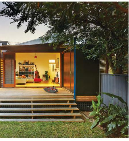
Nairn and Emily were interested in the 'story' of materials and wanted to reuse as much as possible during the renovation, so had stockpiled various things over the years. The tensioned awning used over the deck is braced by welded steel sections from the former lift structure of the Great Northern Hotel.
