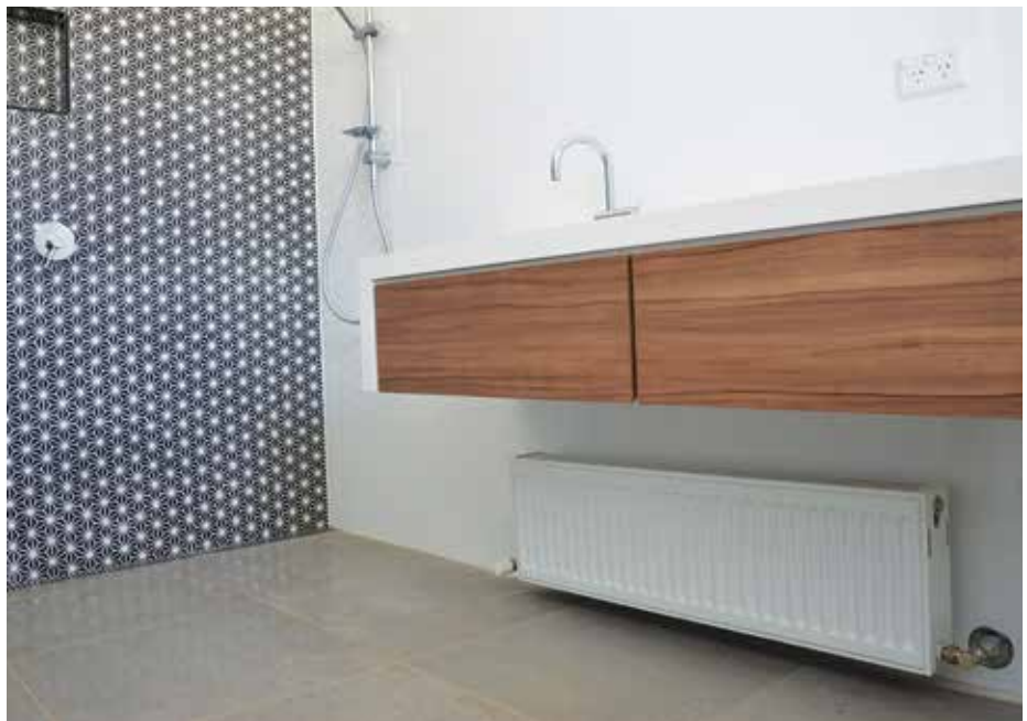
A wall-mounted hydronic radiator panel.
