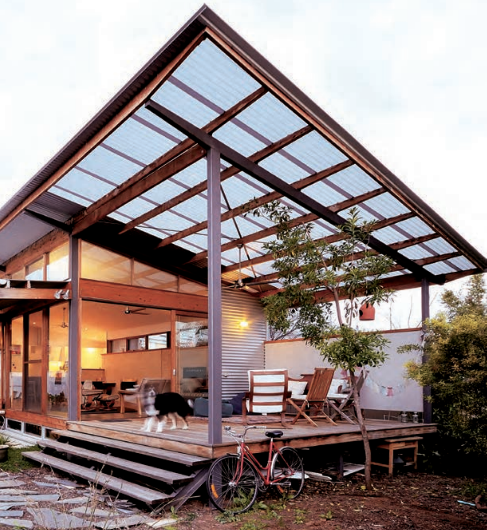
The long, slim extension maximises northern light to make the most of the benefits of passive solar design. Keeping the building's footprint small also maintained a generous and much-loved backyard with room to grow vegetables and space for the kids to play.
