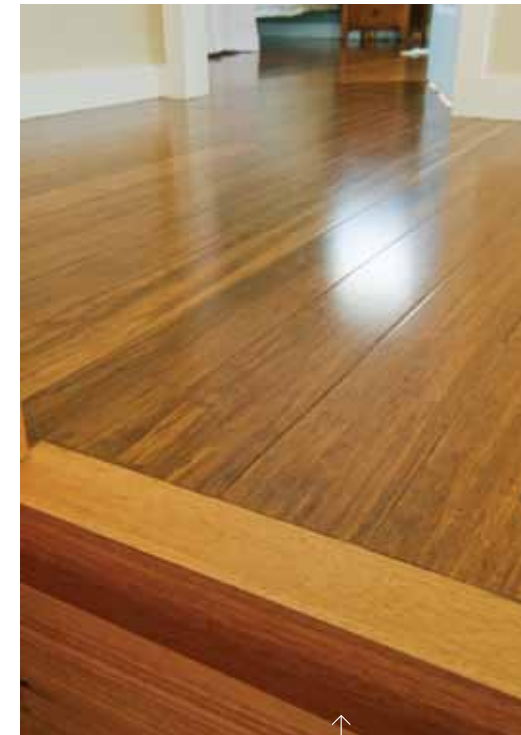
Strong and durable strandwoven bamboo is used for the flooring of the upstairs room.
