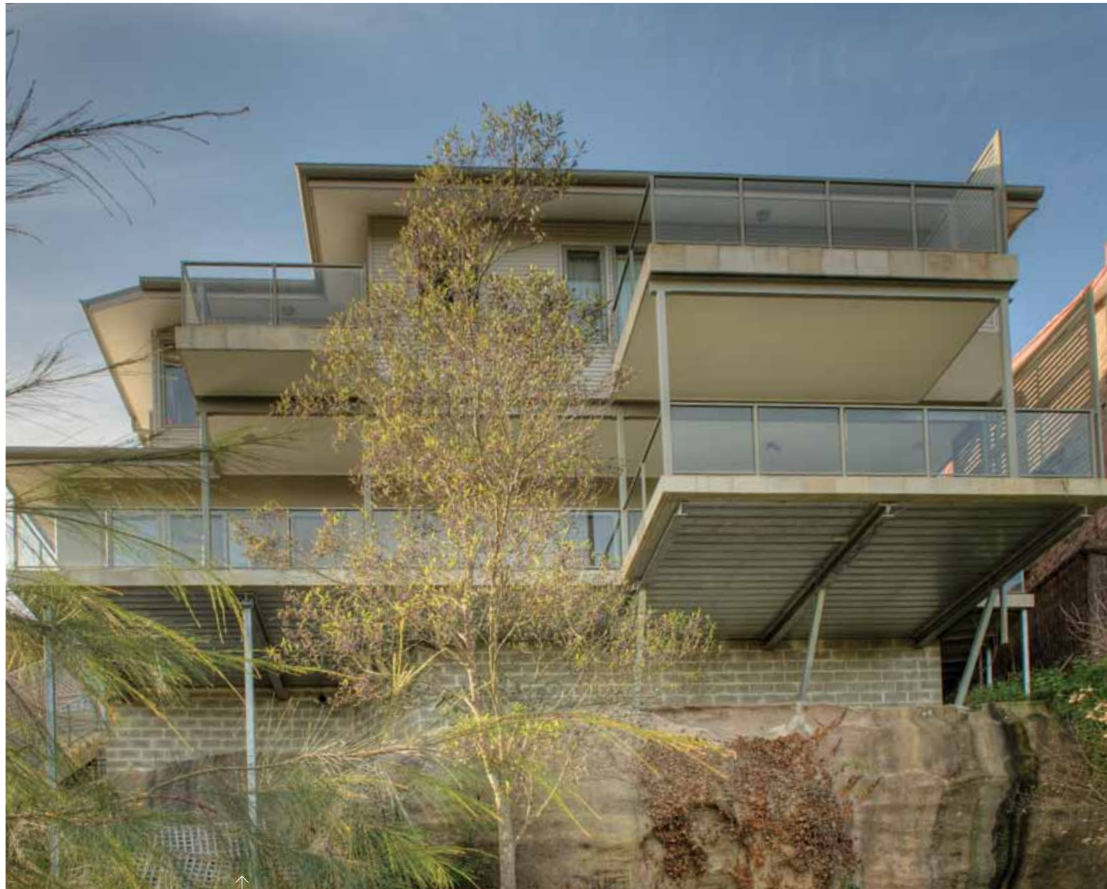
The house is perched at the edge of a six-metre sandstone platform with balconies cantilevered out into space to capitalise on the beautiful views to the south.
