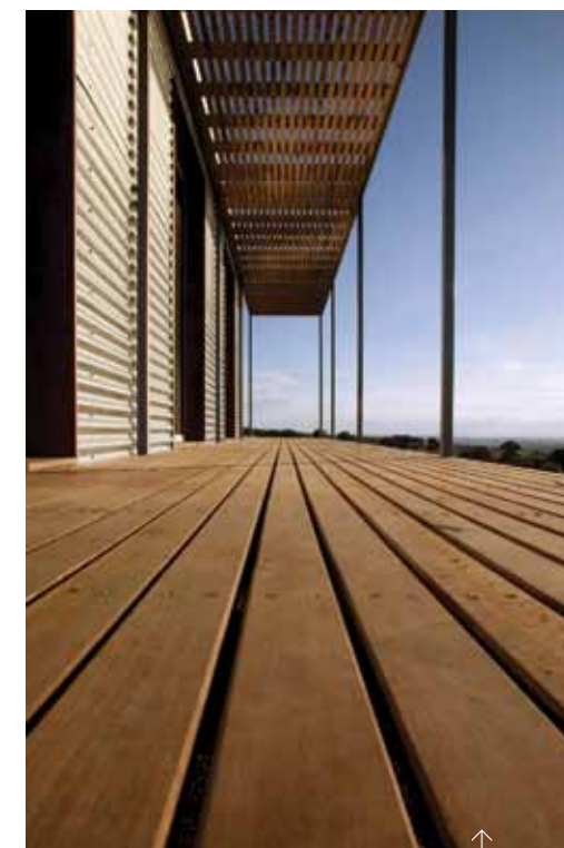
The house is surrounded by wide expanses of spotted gum decking, which lead the eye to the magnificent views.
