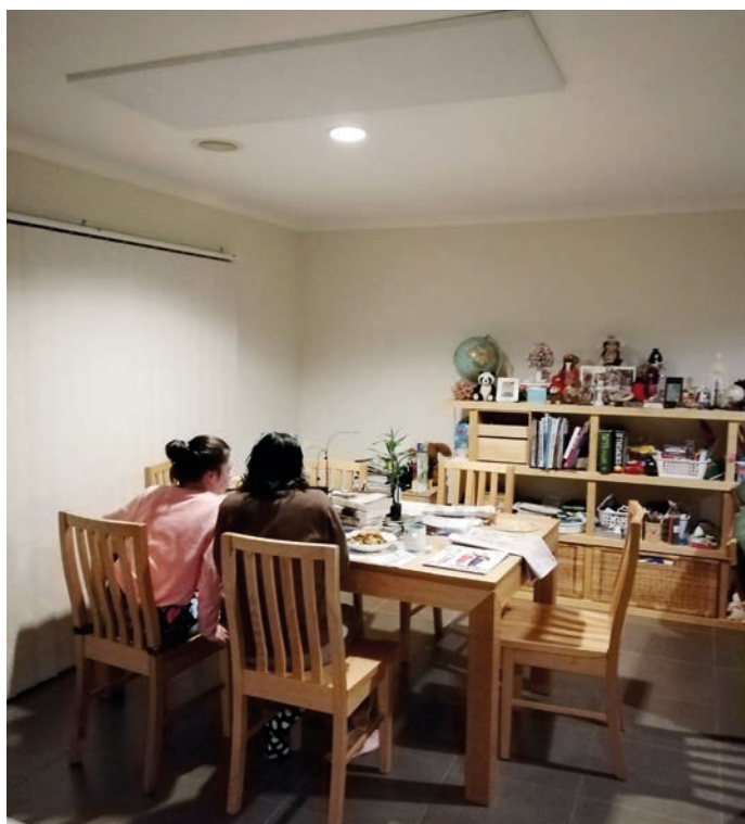
← The far infrared heating panel on the ceiling above the dining table.
