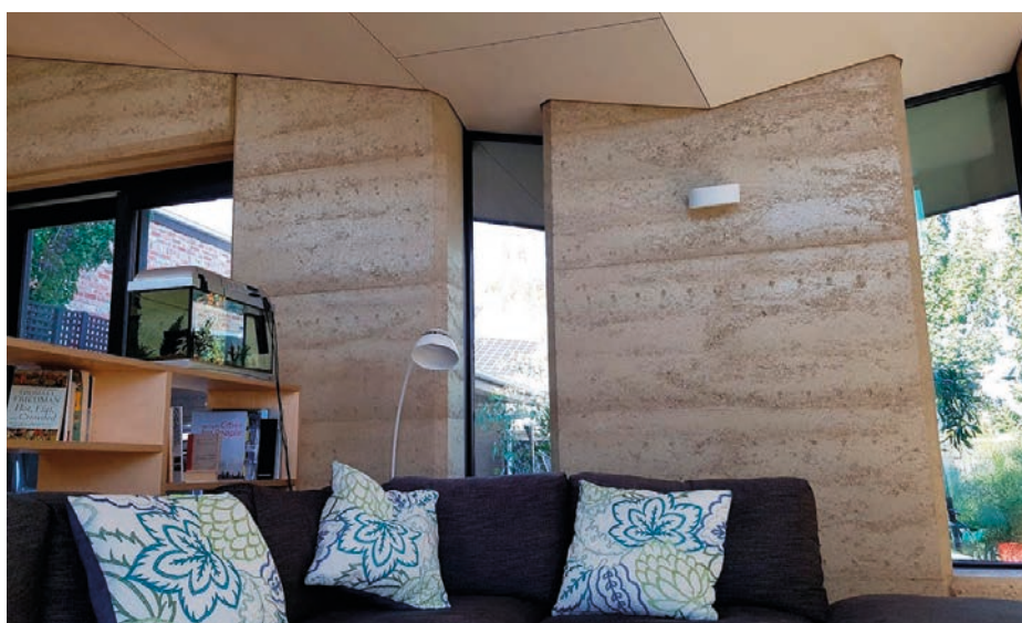
↑ The rammed earth wall is one of the high-performance features of Cameron's home, providing thermal mass to moderate internal temperatures. They've been monitoring how it performs (see Figure 6).
