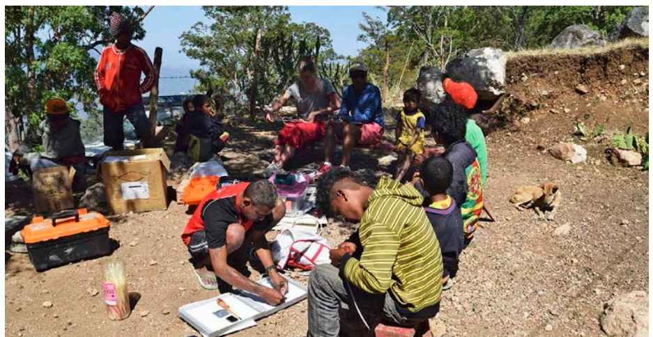
↑ Pre-wiring activities at our village base outside the eating and sleeping hut. Technicians and team members all pitched in.
