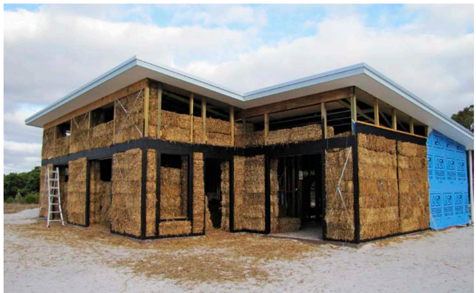
↑ Strawbale walls can have a wooden frame, or can be load bearing. The bales are fitted and rendered to seal them from moisture and vermin.
