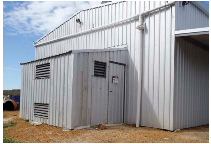
↑ The energy system is contained in a separate room at the end of the Shouse.
