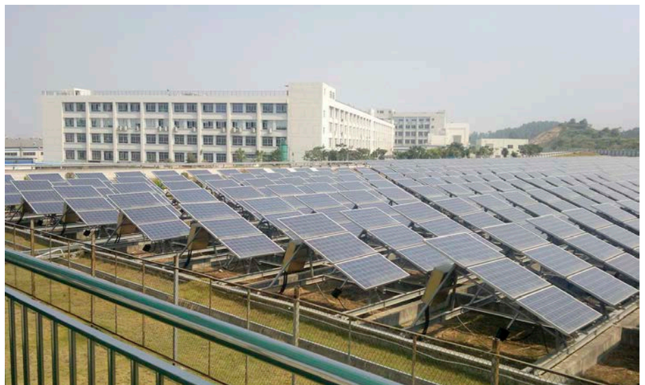
↑ Some solar factories are more like cities than factories. This company employs 180,000 people, with 40,000 just at this one factory, and has built its own 1 megawatt solar installation for panel testing!
